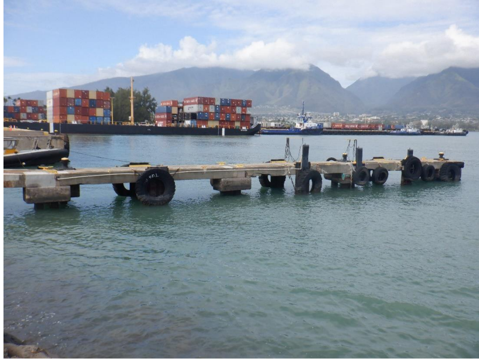
Photo 3: Existing Fender System at Tug Pier
